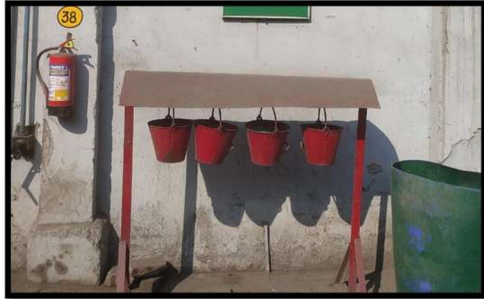
Photograph showing Fire safety equipment
