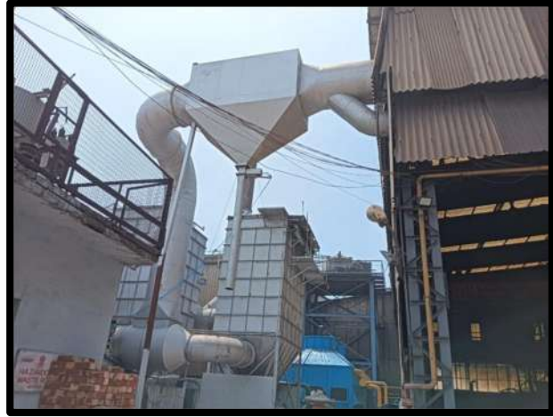
APCD installed in project premises
