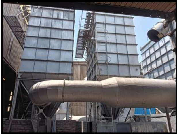
APCD installed in project premises
