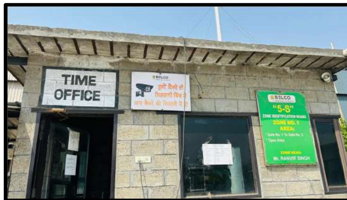
Photographs showing project premises and Env. Data board
